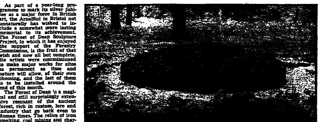
David Nash's Black Dome under construction in the Forest of Dean
